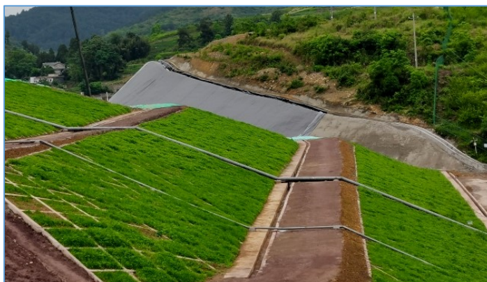
Figure 7. Application of ecological remediation technology for bauxite residue-based soil.
